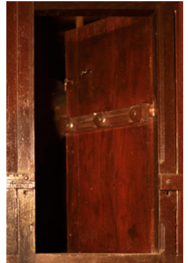
The door of arra. In traditional Kerala agrarian houses, the central part of the house was a secure wooden granary called arra to store paddy grains until it could be sold. It was rodent proof and raised several feet above ground level to avoid flooding during the monsoons.
