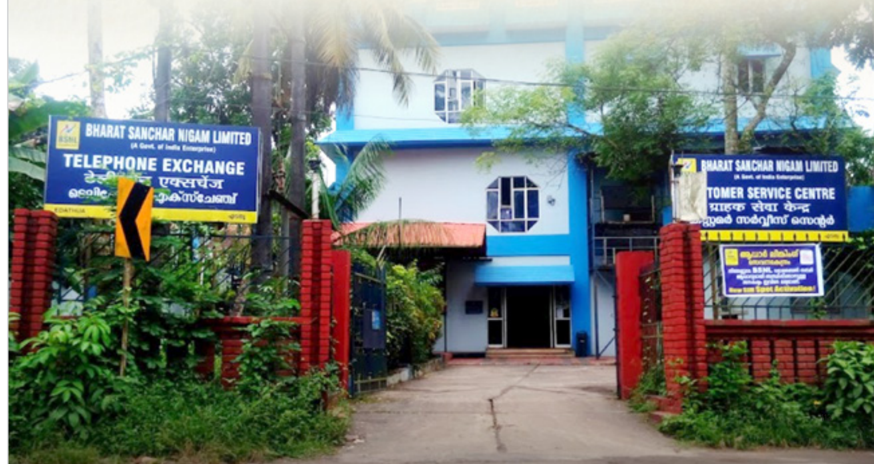
Edathua Telephone Exchange.
